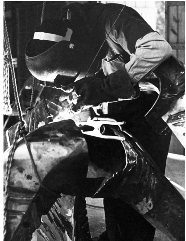
Several weeks after the various segments are cleaned and the welding process begins.
